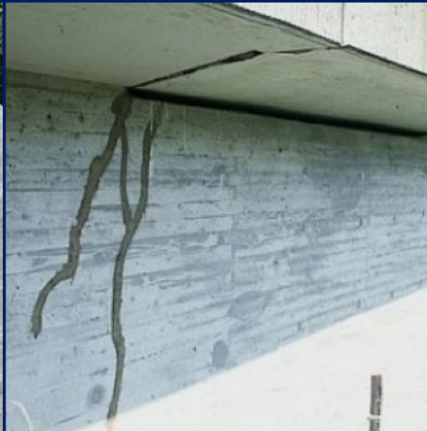
Detection of cracks
