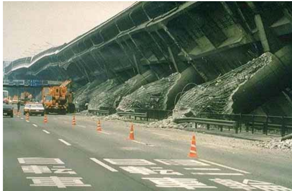
Hanshin Expressway Bridge after Kobe earthquake, Japan, 1995.
